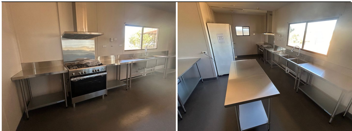
Golf Club Upgrade Stage 1 – Plumbing Works and Kitchen Upgrade
